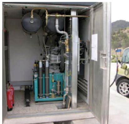
*Compression equipment (left) and refuelling station (right)*
