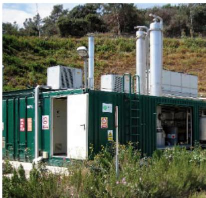
*Biogas upgrading plant*
