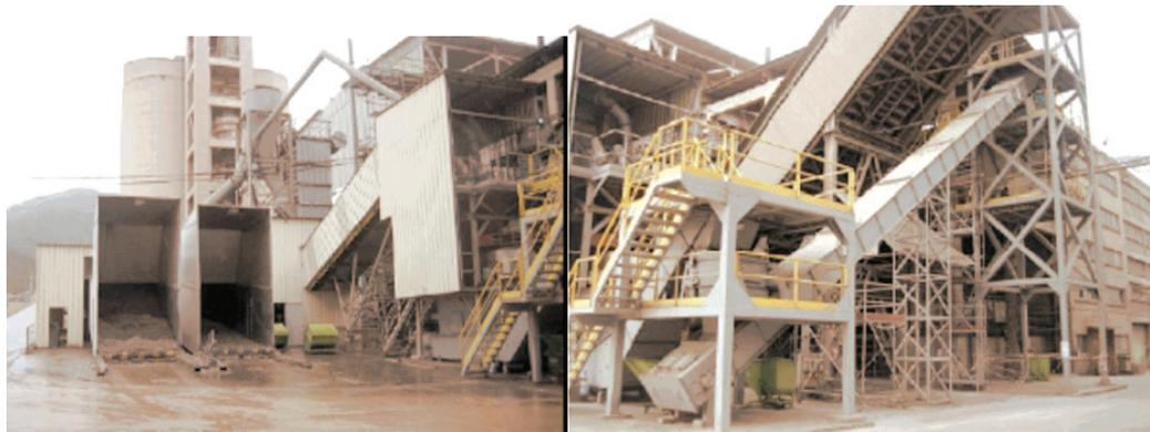
The facility is located close to the cooling satellites of furnace number 3. The installation is comprised of two mobile storage units, bag filters, material transport conveyors, screening and scale metering and a pneumatic conveying system (airlock and blower to the oven's burner).
