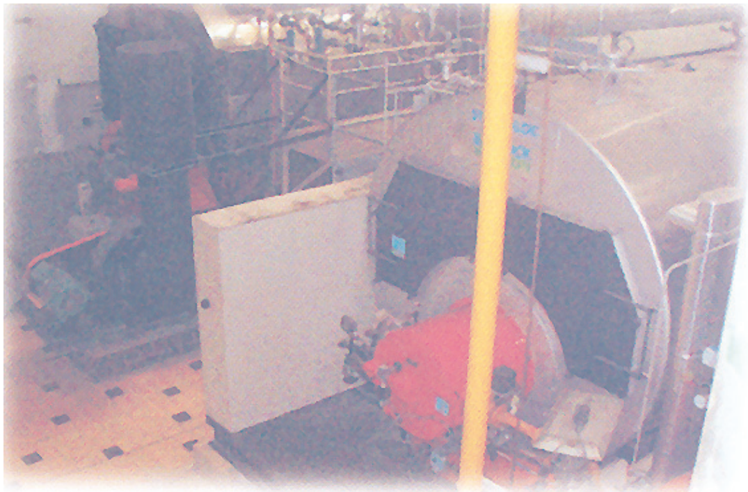
Boiler in the cheese production process
