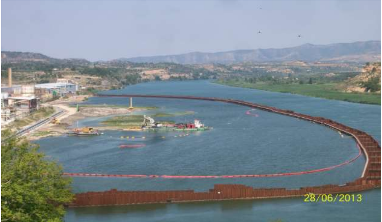
Dredging activities inside the sheet piling
