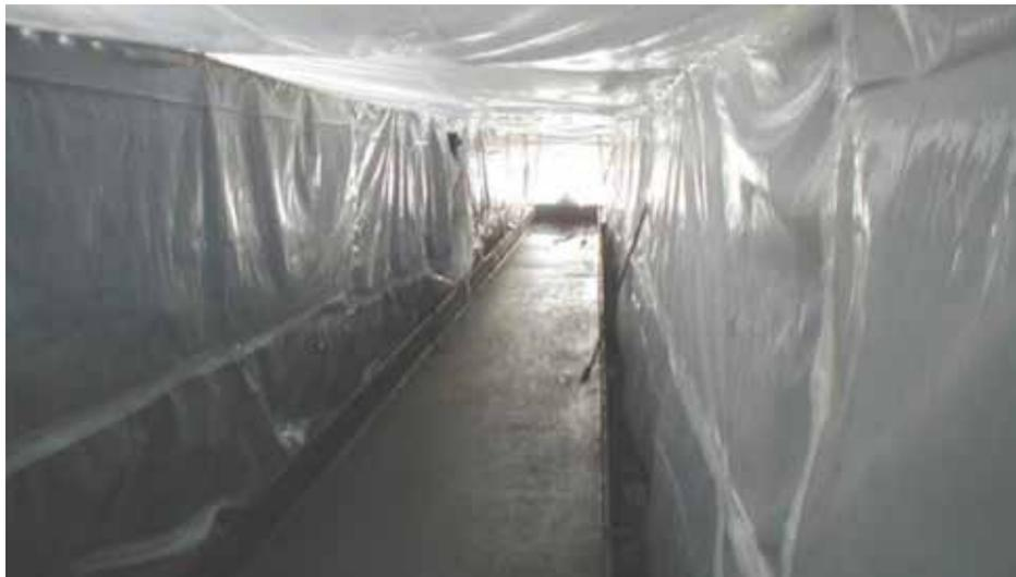
*Cell confinement (connected to the air treatment unit)*
