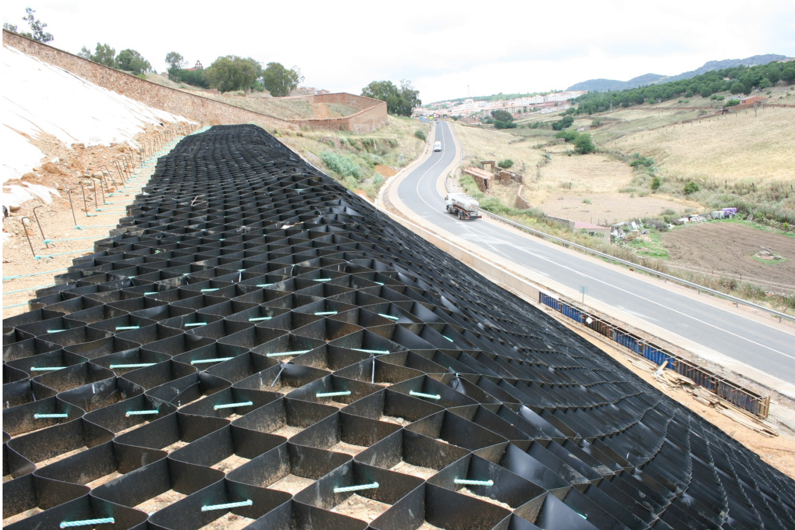
GEOCELLS SOUTH SLOPE
