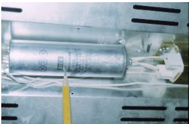
Figure 2. A typical PCB-capacitor, inside a lighting fixture.
