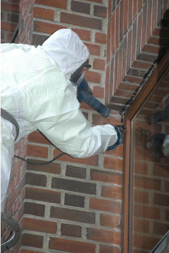
Figure 7 Removal of sealant around a window.
