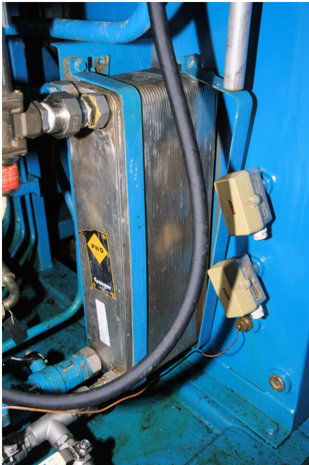
Figure 5 This is a modern heat exchanger (labeled "PWO"), but we assume old ones look similar to this.
