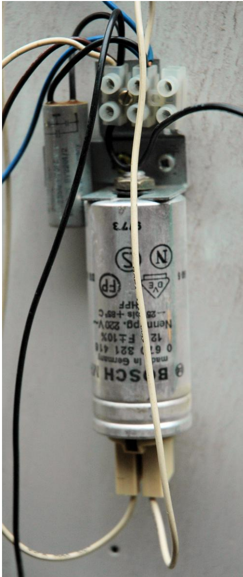
Figure 1. Typical aluminum can capacitor, might contain PCB.
