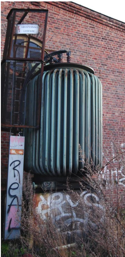
Figure 9 Typical PCB-containing transformer.
