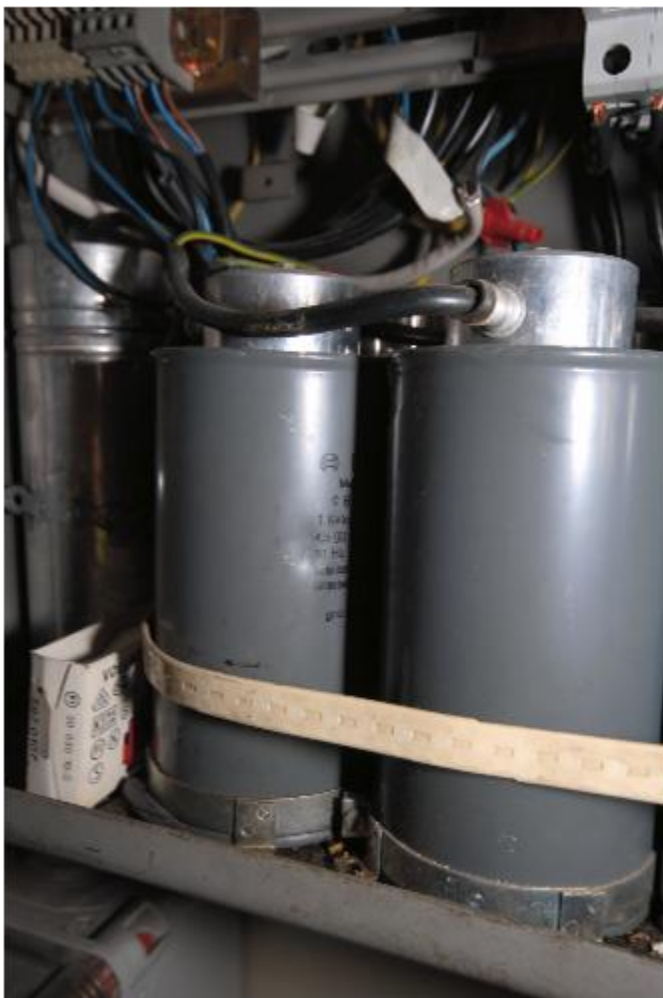
Figure 1 Here you can see PCB-capacitors in a fuse box.
